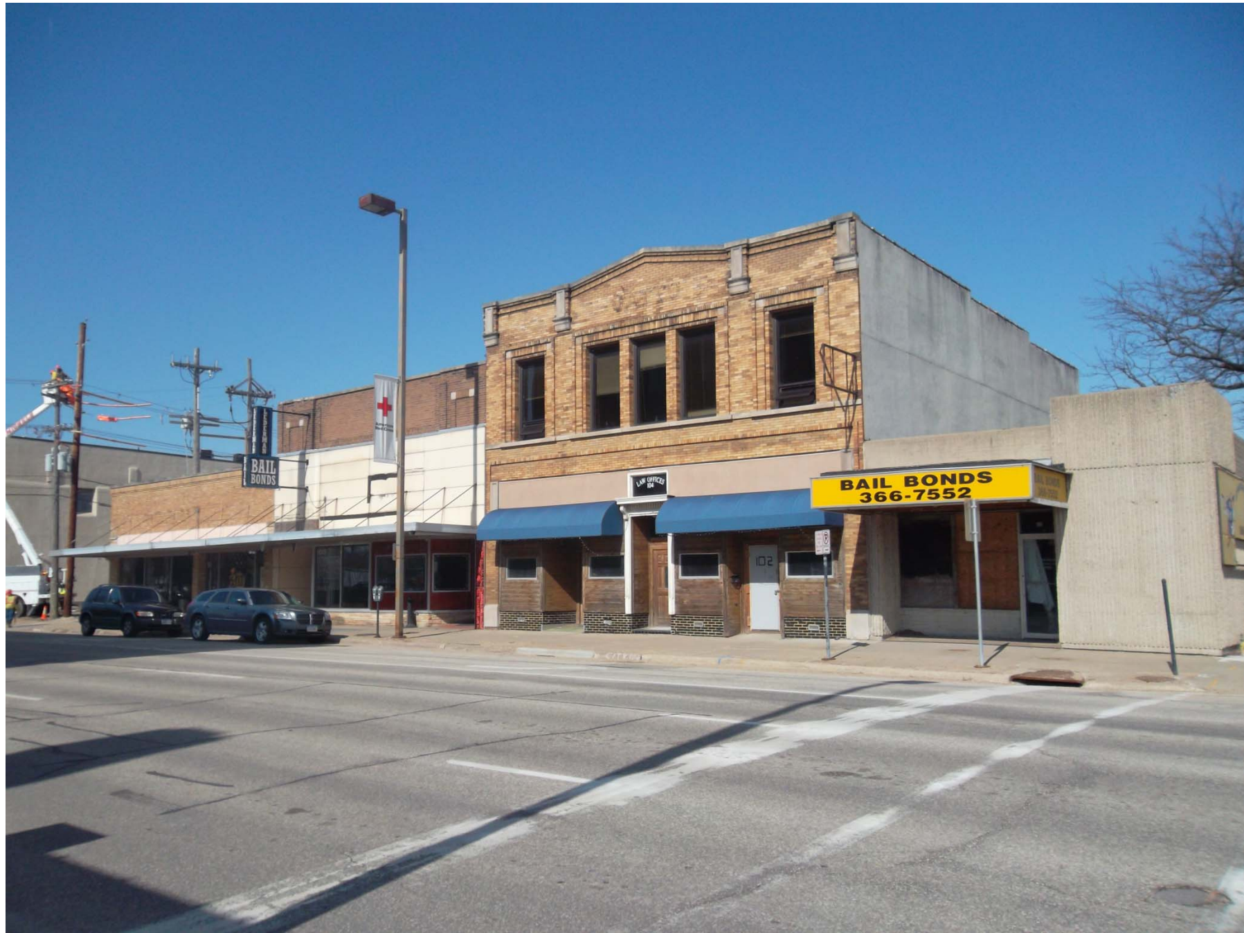
Photo 1 of 13. 3 rd Avenue SW, North side of street, looking northwest.
