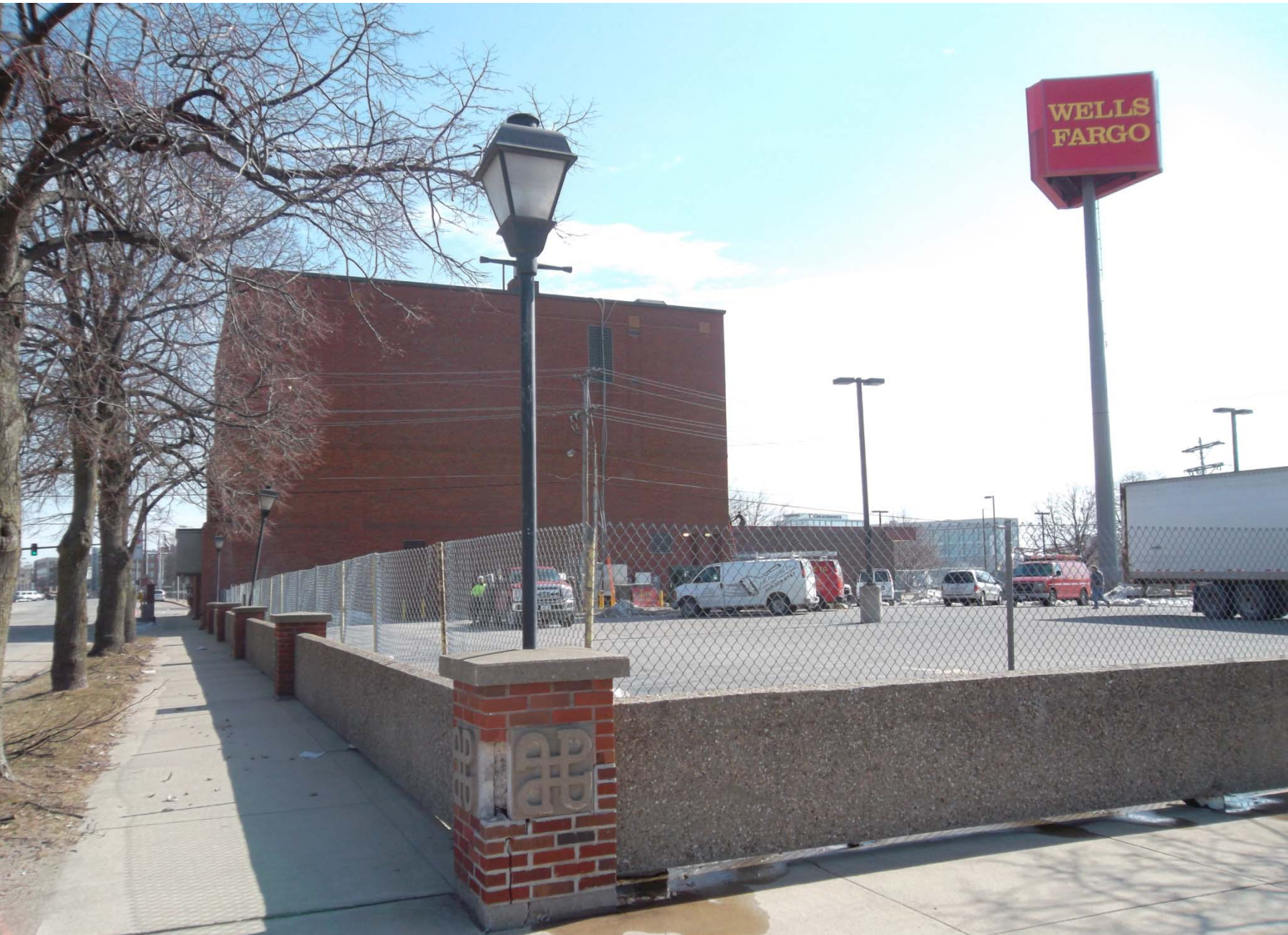
Photo 10 of 13. 3 rd Avenue SW, South side of street, looking northeast.
