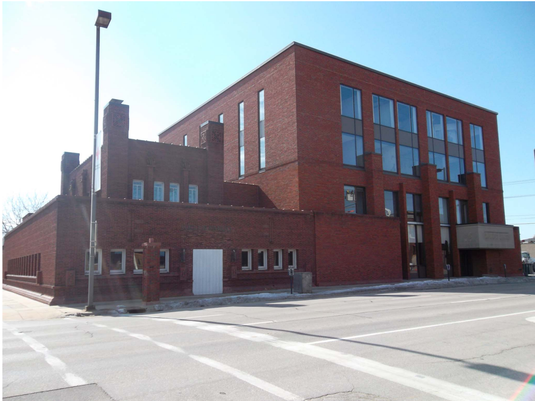
Photo 12 of 13. 3 rd Avenue SW, South side of street, looking southwest.
