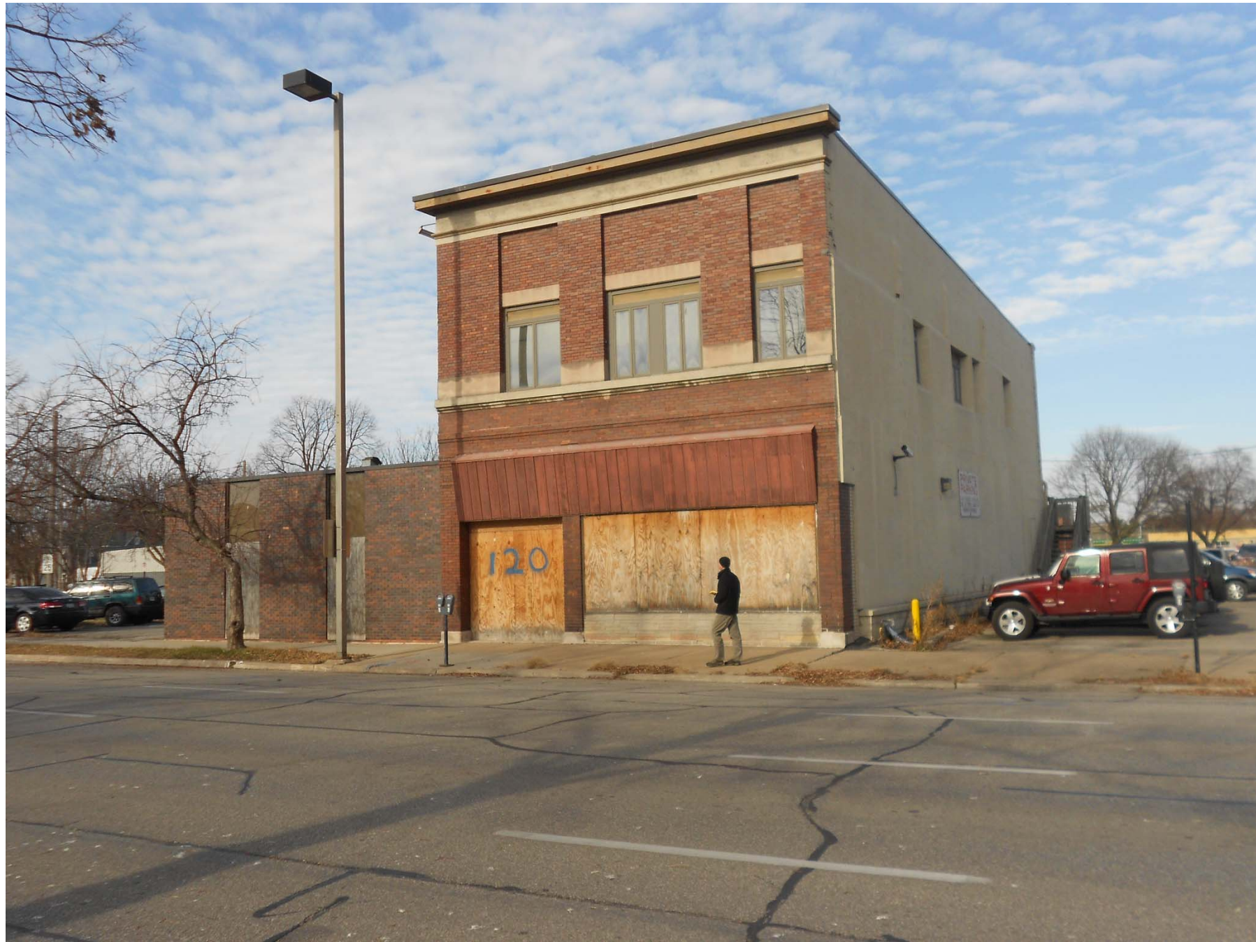
Photo 3 of 13. 3 rd Avenue SW, North side of street, looking north-northwest.
