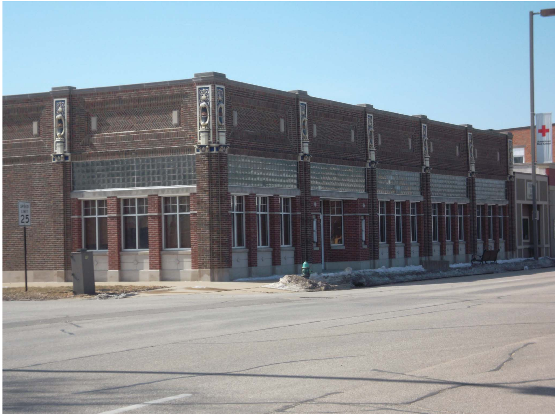
Photo 9 of 13. 3 rd Avenue SW, South side of street, looking southwest.
