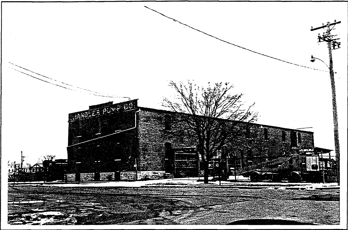
Chandler Pump Company
