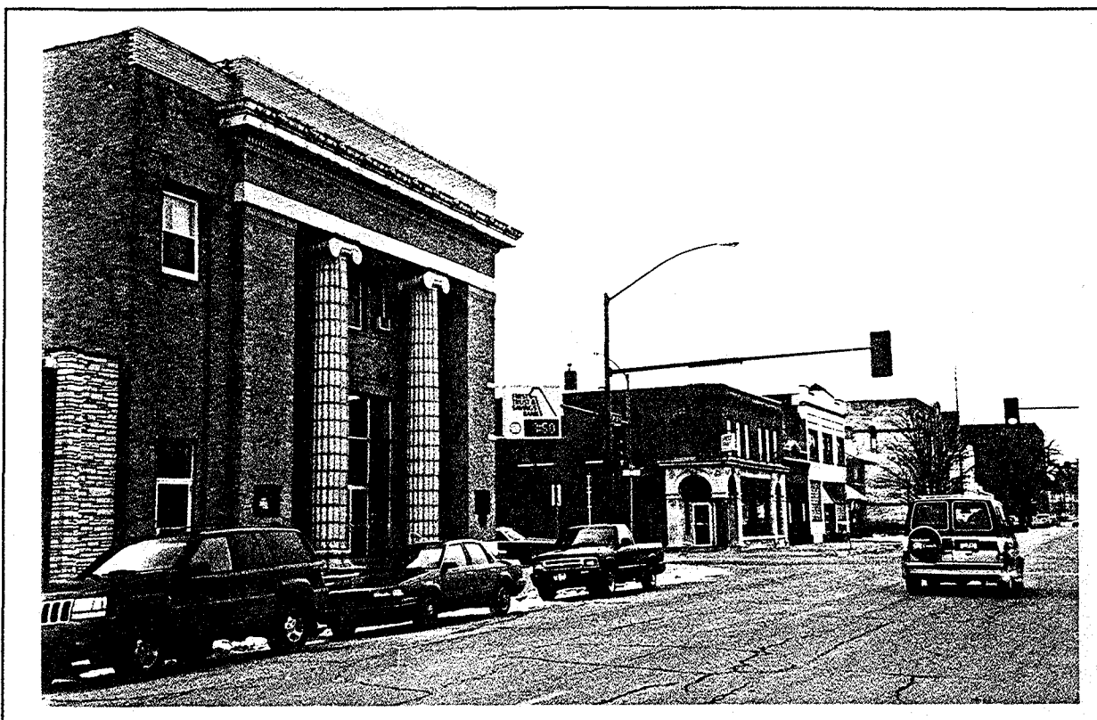
Iowa State Bank, 1917 building, left, and 1906 building, center; 3rd Street, SE and 12th Avenue, SE
