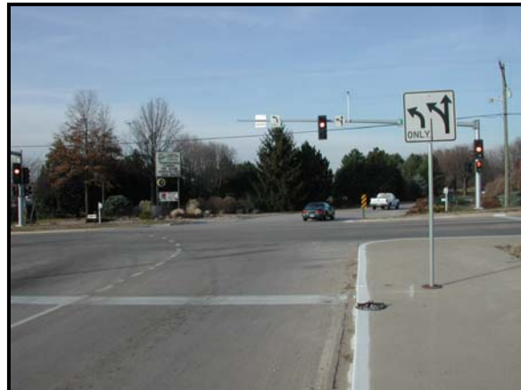
Edgewood Rd looking northbound
