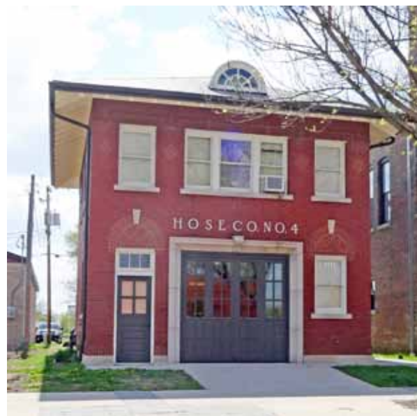
Figure 41: Hose Company #4 rehabilitation at 1111 Third Street SE in the Bohemian Commercial Historic District. Built in 1915.
