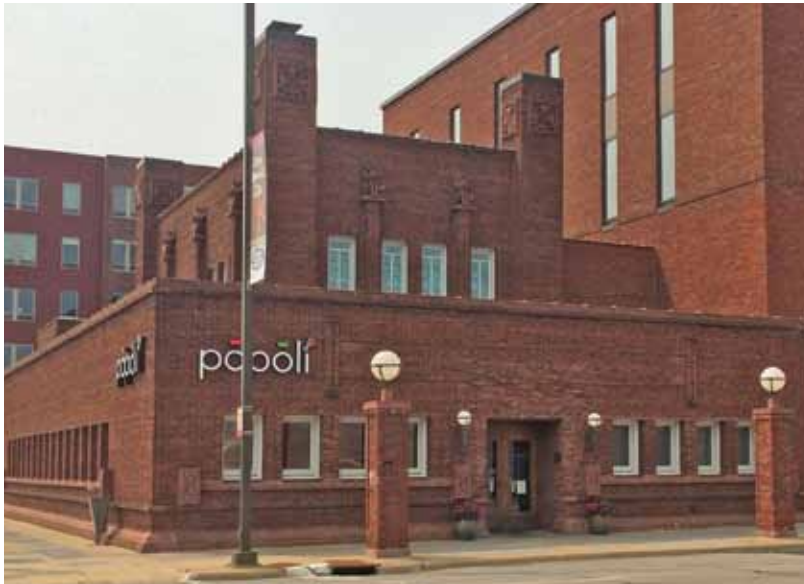
Figure 94: Peoples Savings Bank (Popoli's Restaurant) at 101 Third Avenue SW was designed by architect Louis Sullivan (1910-1912).
