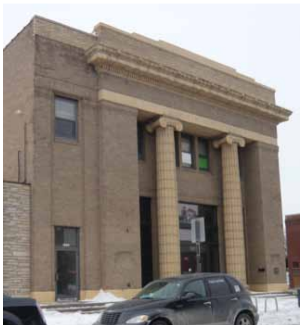
Figure 89: Iowa State Savings Bank (1917) at 1201 Third Street SE.
