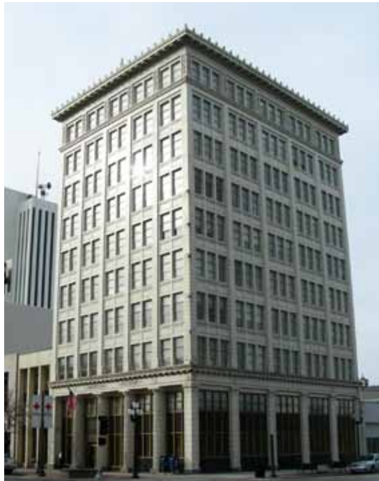
Figure 93: American Bank Building (1913-1914) at 101 Second Street SE.
