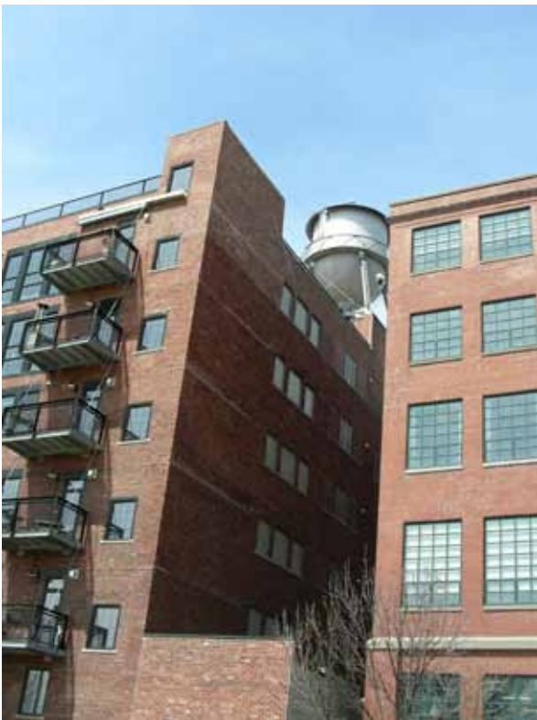
Figure 73: Left: Churchill Drug Wholesale Building (1925) (Water Tower Place) at 900 Second Street SE. Right: Witwer Grocer Building (1946) (NRHP) (Bottleworks) at 905 Third Street SE.
