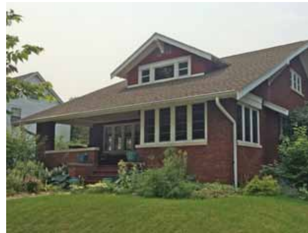
Figure 79: Many buildings such as this employed the Craftsman style in one fashion or another.
