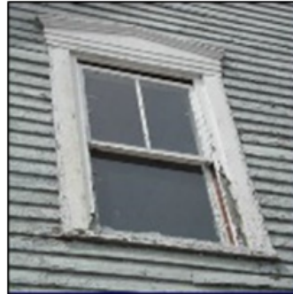
Repairable historic window
