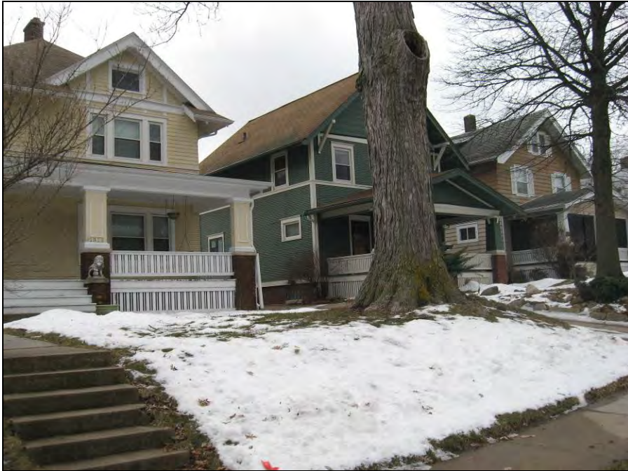
East Highlands: 1323 through 1331 Third Avenue SW, facing south.
