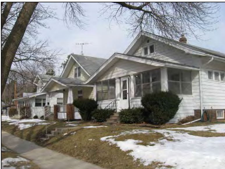
North Highlands: 1730 through 1722 B Avenue NW, facing northwest.
