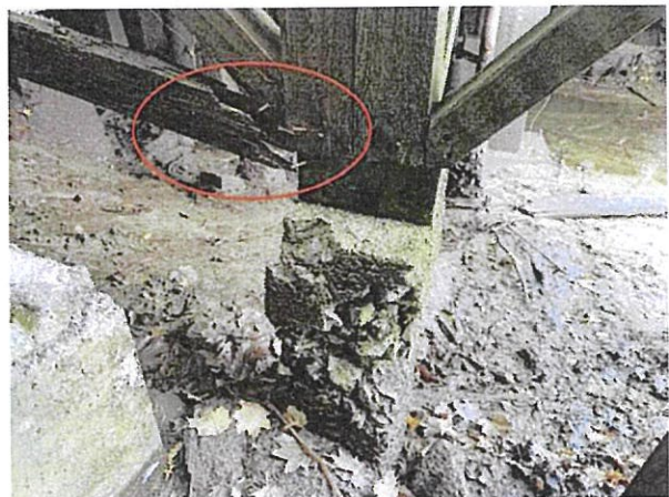
Photo 20: Broken brace
