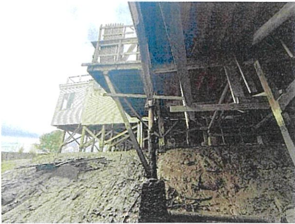
Photo 5: Typical floor and foundation framing
