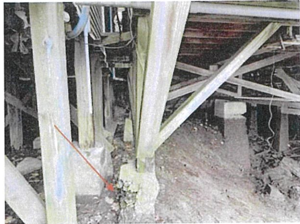
Photo 12: Deteriorated foundation piers
