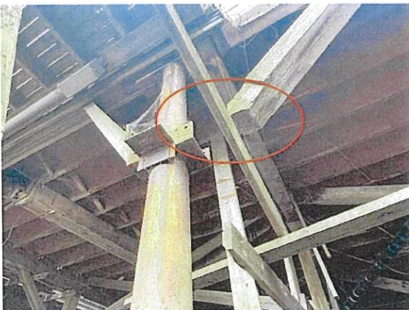
Photo 19: Broken brace
