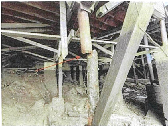
Photo 7: Corroded steel foundation post
