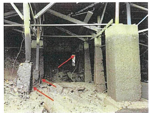
Photo 10: Out-of-plumb concrete foundation piers
