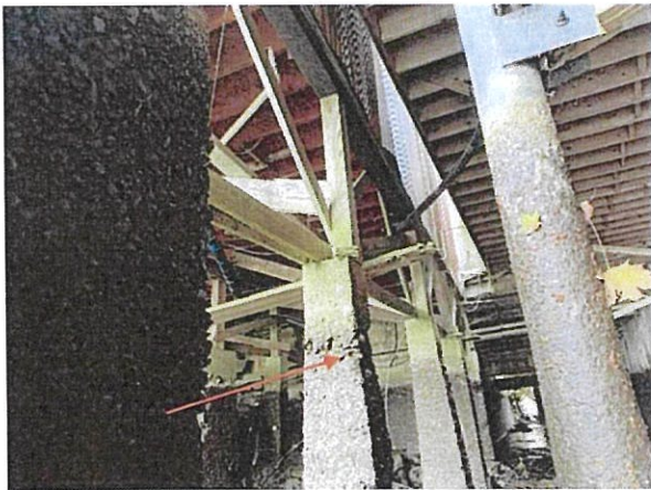
Photo 13: Deteriorated foundation piers
