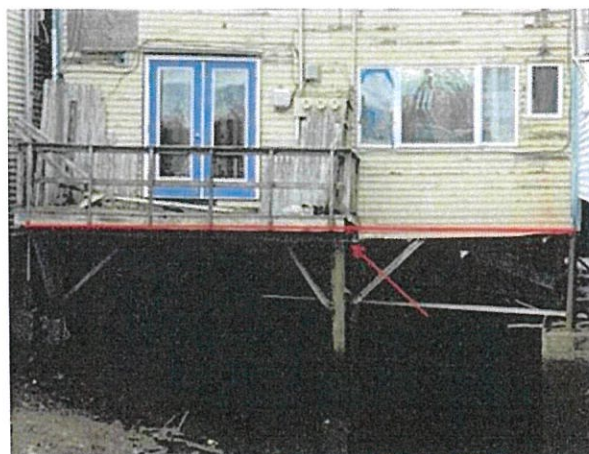
Photo 9: Sagging floor structure at corroded post
