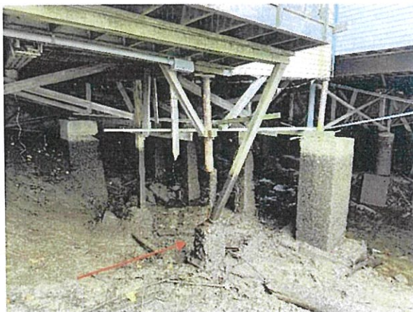
Photo 15: Deteriorated foundation piers
