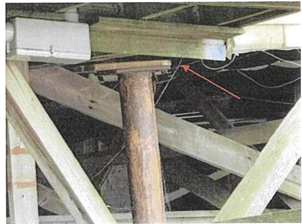
Photo 8: Steel post not attached to the structure
