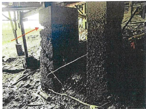
Photo 14: Deteriorated foundation piers
