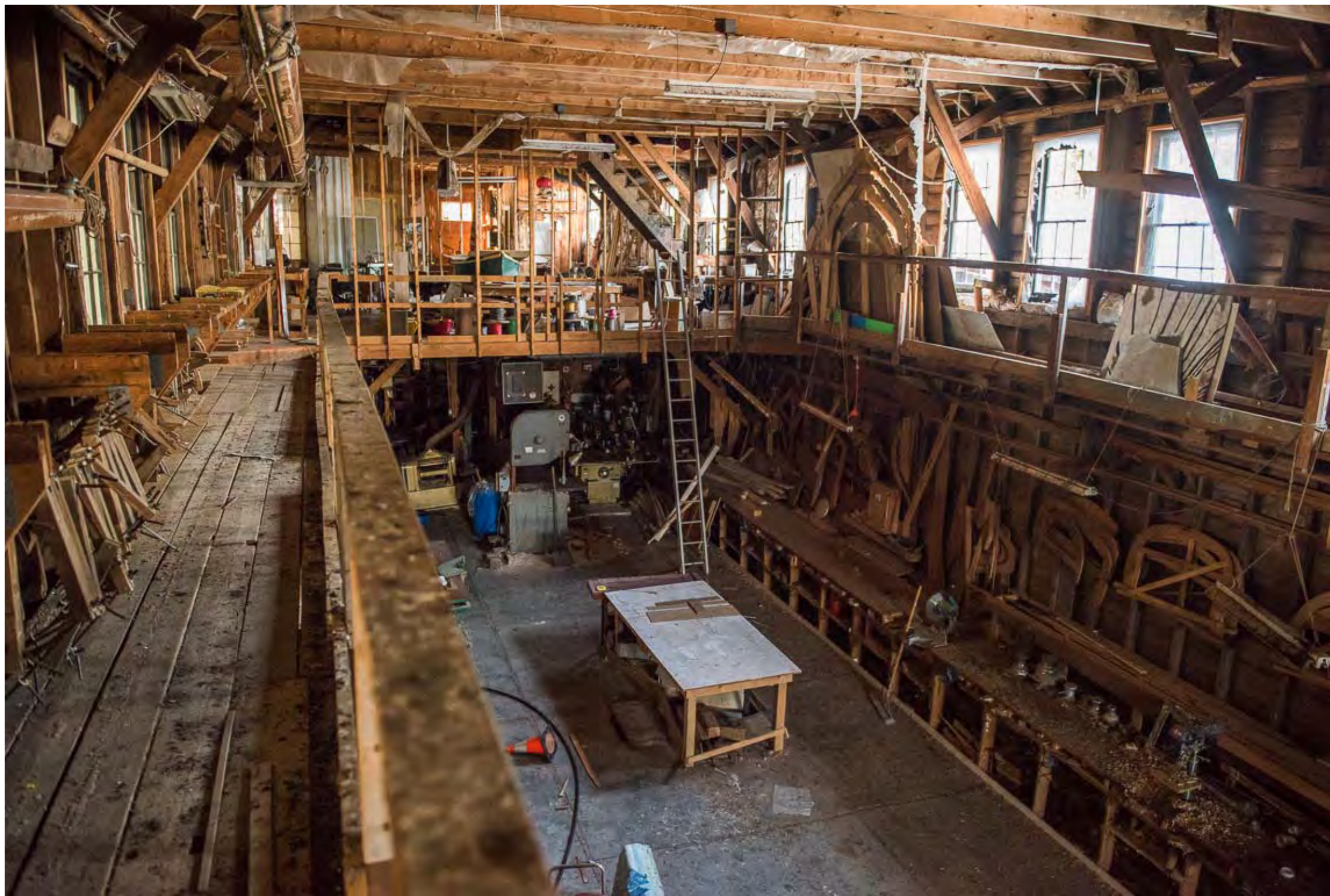
INTERIOR EXISTING CONDITIONS IMAGES American Boat House 17 Atlantic Avenue, Camden
