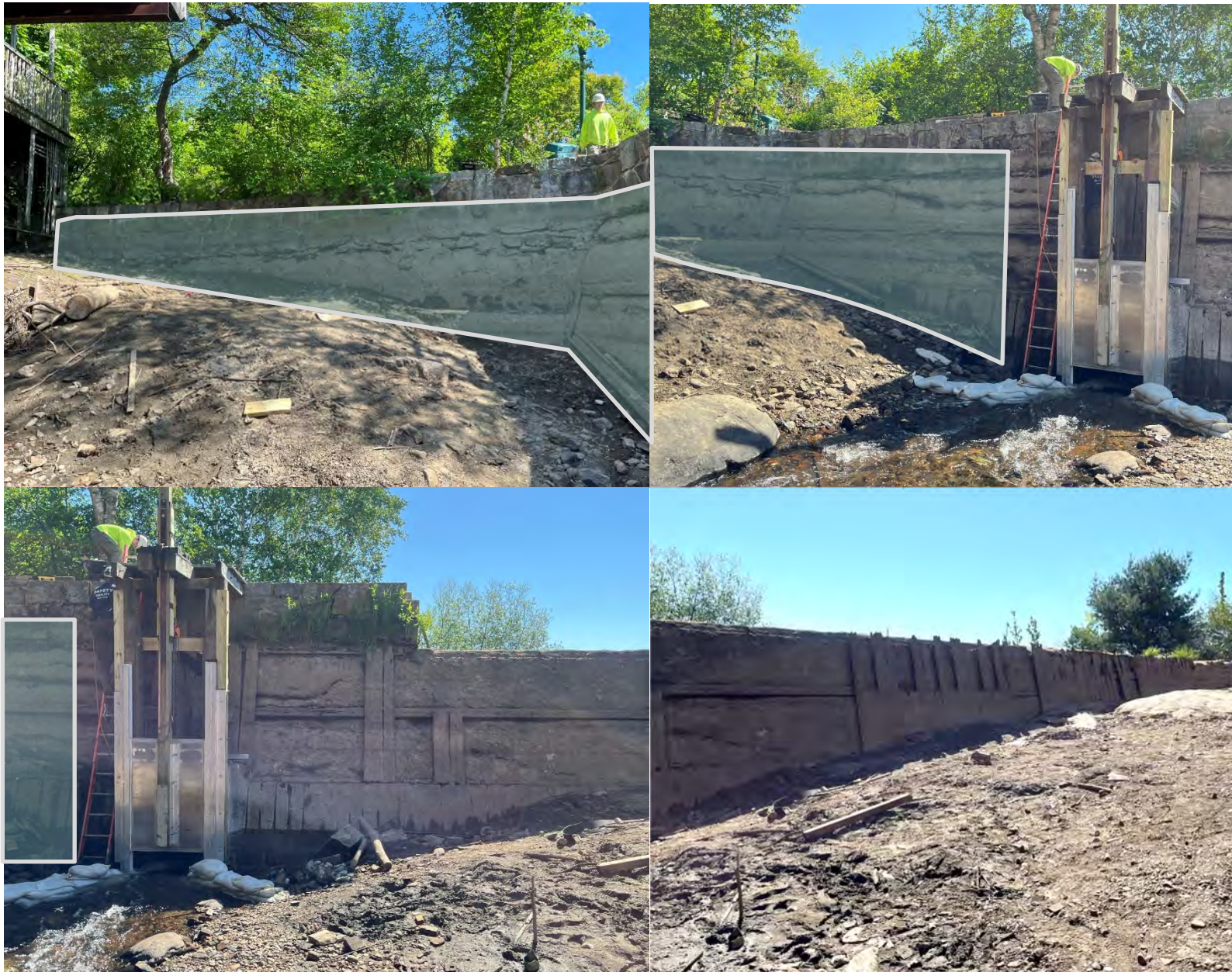
Figure 2: Interior of Dam for north (upper left) to south (lower right) with Conceptual Concrete Overlay Area shaded. Other areas would be reconstructed.
