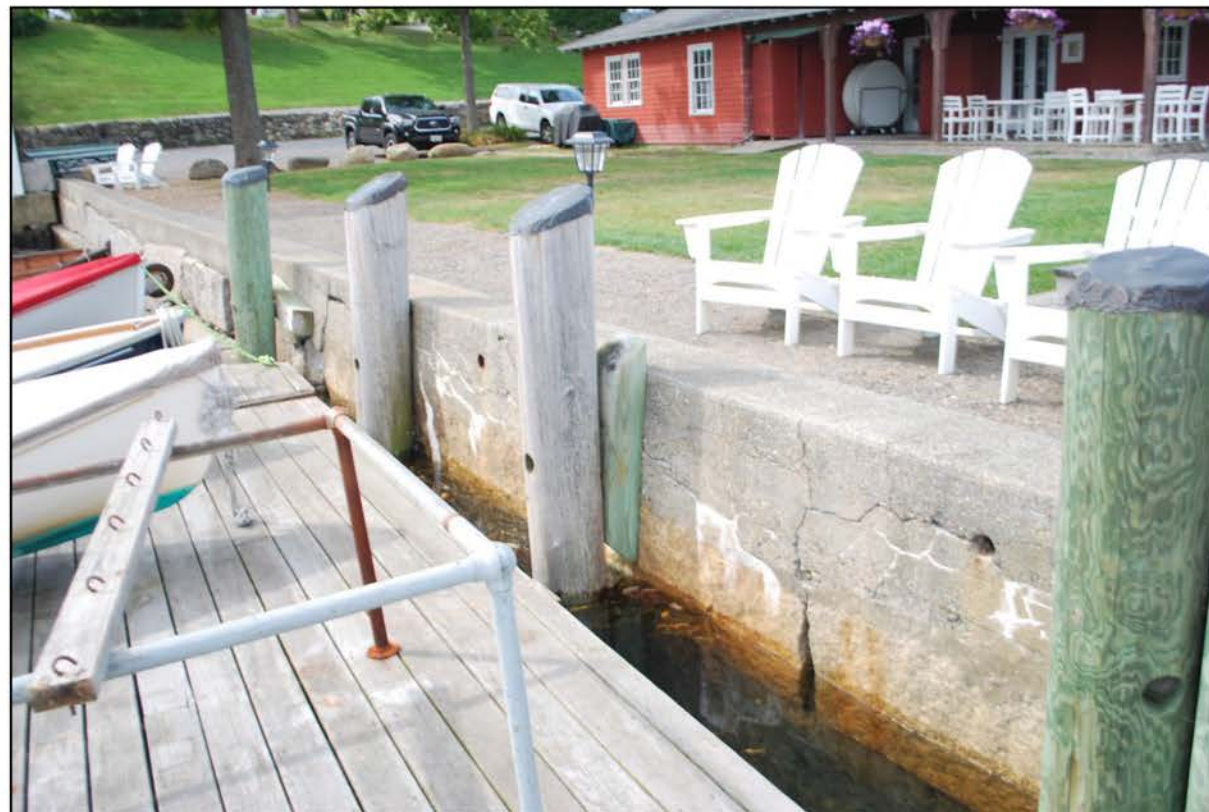
Photograph 30: Camden Yacht Club stacked granite seawall and concrete cap with fresh fill behind.
