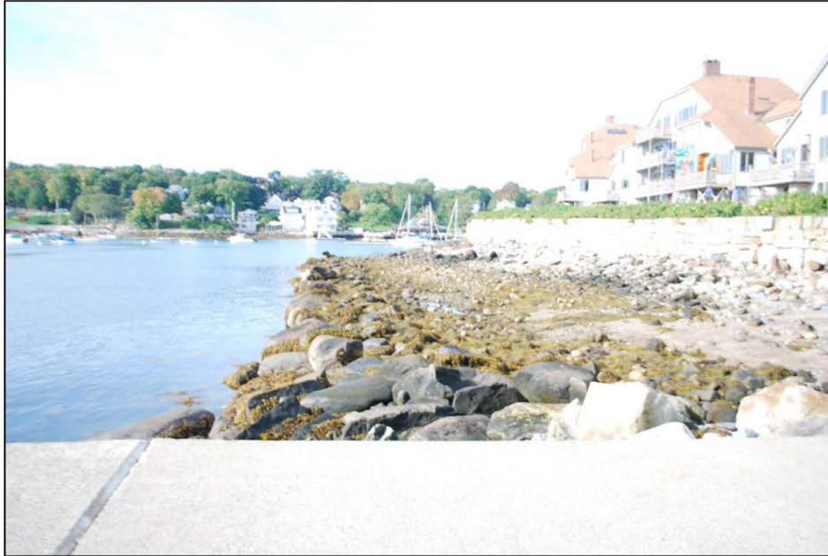
Photograph 1: Offshore seawall in front of townhomes stacked granite seawall.
