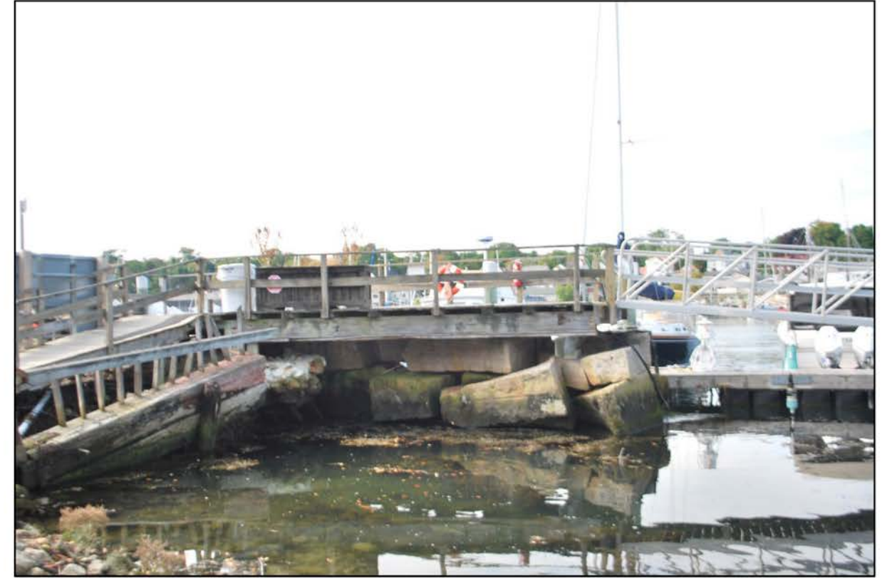
Photograph 11: Displaced stacked granite at north end of Lyman Morse Wharf.
