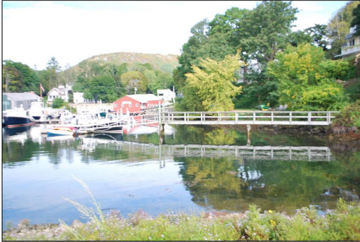
Photograph 13: Timber pier with gangway and float extending from private property.
