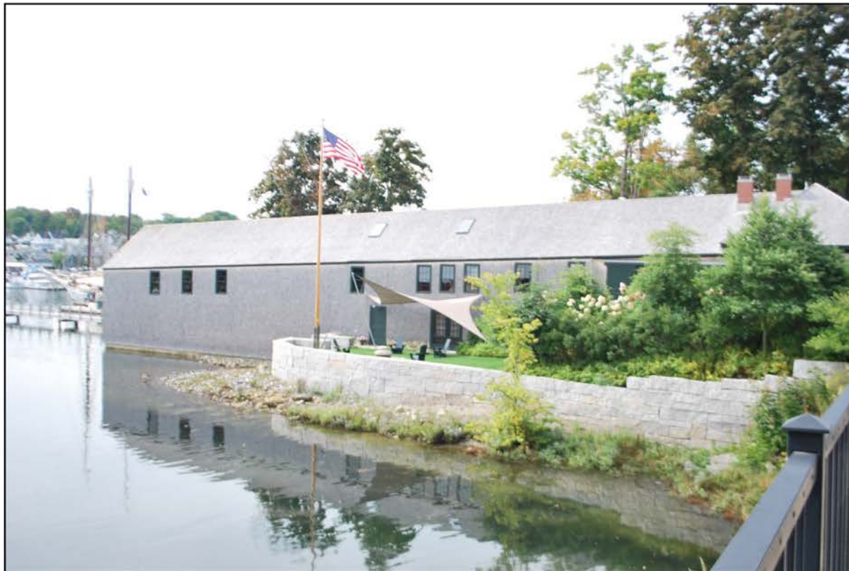
Photograph 18: New stacked granite seawall with American Boathouse in background.
