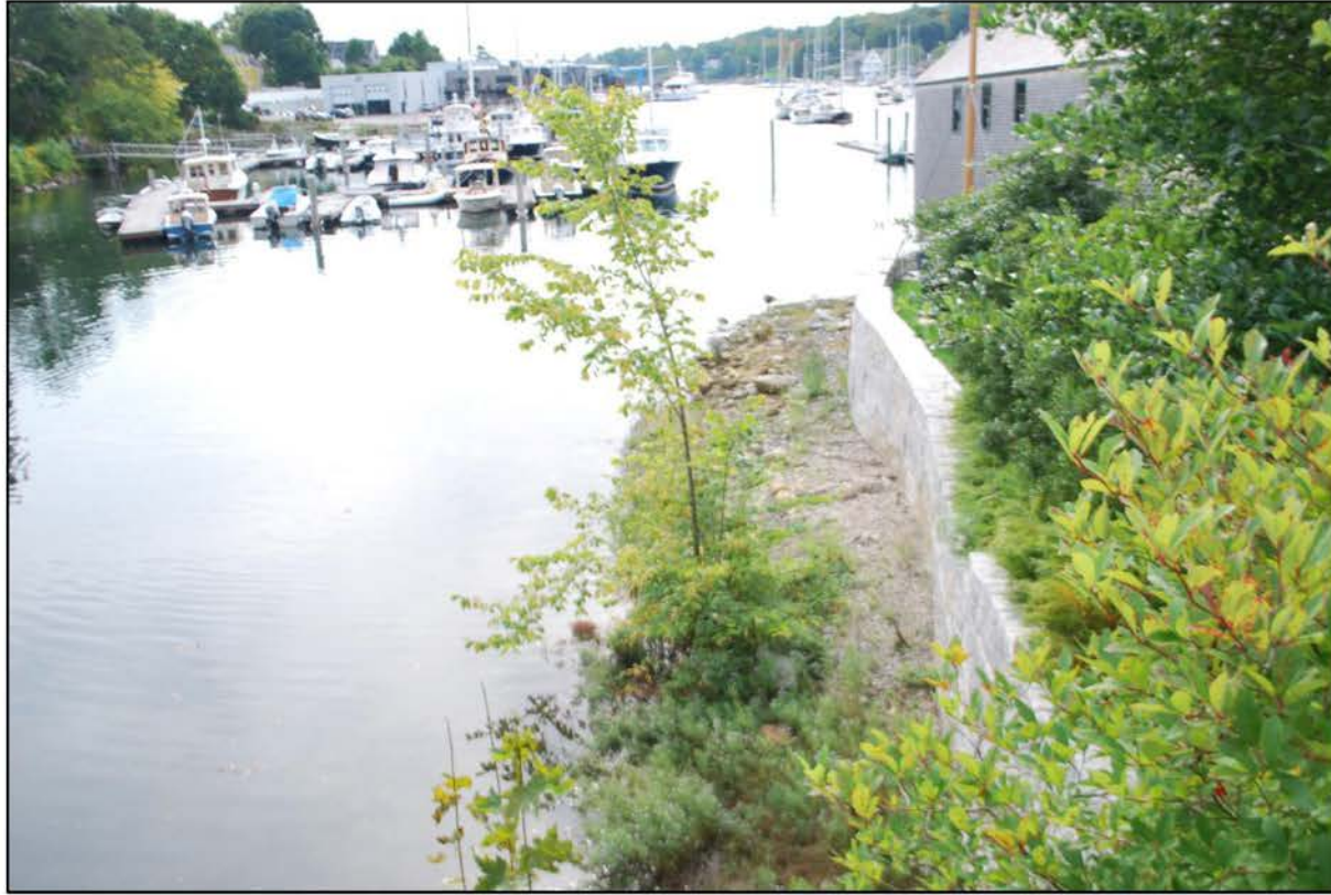
Photograph 17: New stacked granite seawall at American Boathouse.
