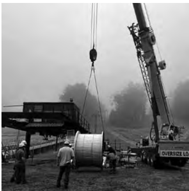
The triple chairlift cable replacement project demanded a lot of coordination, planning and hard work.
