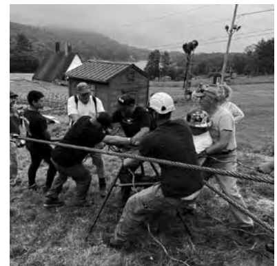
The triple chairlift cable replacement project demanded a lot of coordination, planning and hard work.
