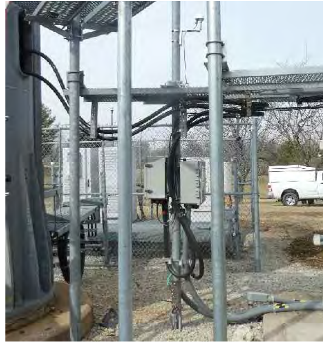
G EXIST. CABLE ROUTE SCALE: NONE
