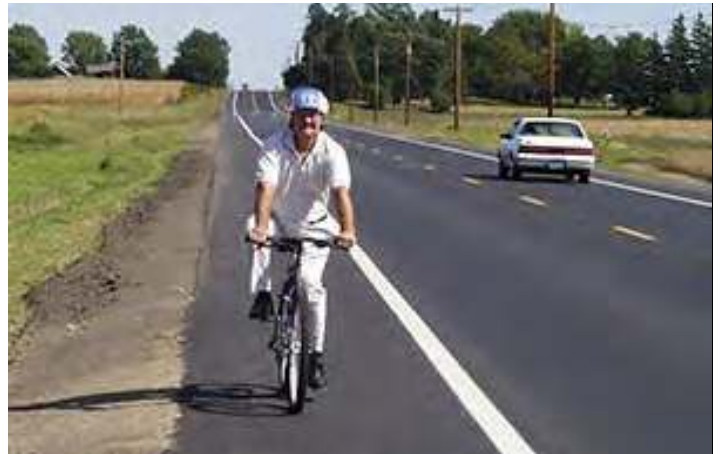
Photo 5: Paved shoulder along roadway
