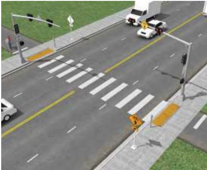
Photo 8: Mid-block crossing with HAWK signal
