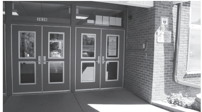
The bond will add additional security in the entrances of all our buildings including enhanced video entry, swipe card access and construction of a two-door entry with a locked vestibule.
