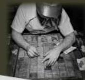
Prior to the 1970s, Linotype machines were used in the production of newspapers. The Linotype output lines of type made from molten metal that were assembled into a form. A New York Times composing room employee is seen assembling a form.
